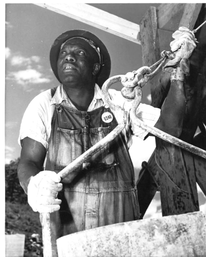
Construction worker at Douglas Dam, TN, 1939 - Courtesy of Library of Congress
