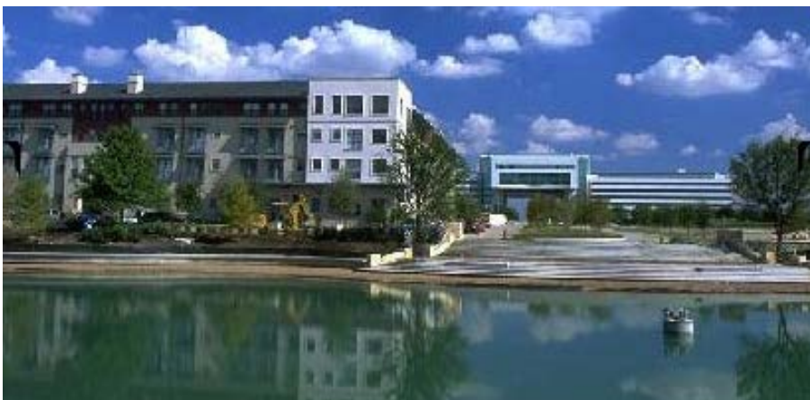
Figure 38. Legacy Town Center in Plano, Texas – a Good Example of Mixed Land Uses, One of the Ten Smart Growth Principles
