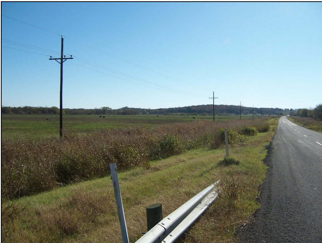
Figure 15. Rural Setting in Fannin County, Texas, North of Dallas
